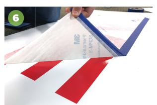
Gently remove the pre-masked transfer tape, starting at a top corner. If any vinyl begins to come off the wall, use your squeegee to firmly adhere it back to the wall and continue peeling away the premask.
