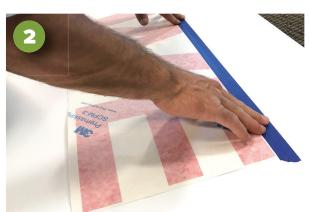
After measuring and marking your intended installation location if necessary, apply a horizontal strip of masking or painters tape to the top of the graphic with the top half of the tape on the intended surface, creating a hinge.
